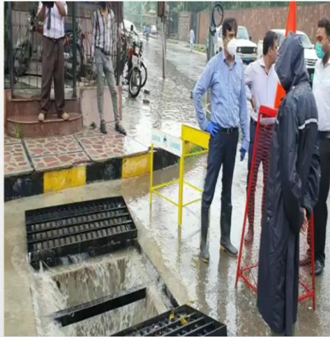
RAINWATER COLLECTION AT RAIN WATER STORAGE TANK
