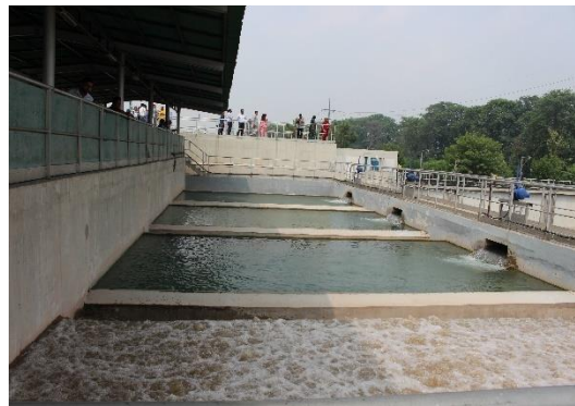
Figure 15:Field Visit of Surface Water Treatment Site
