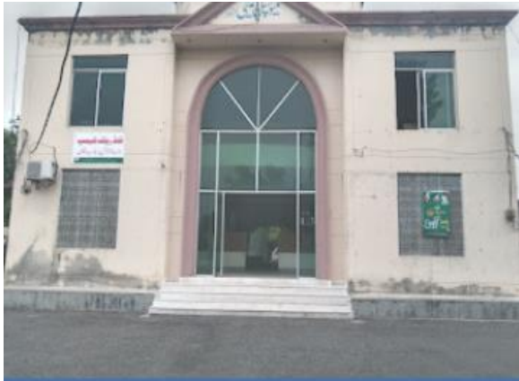
Figure 14: Front view of Main MC Building
