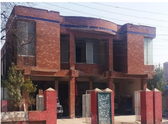
Figure 29: Front view of Fire Brigade
