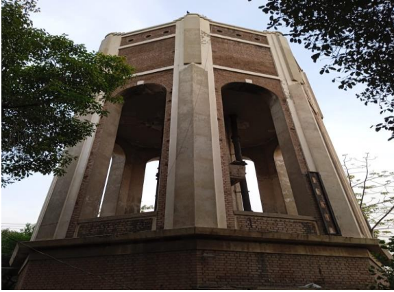
Figure 47: Front View of Water Supply Branch
