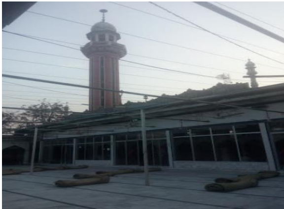
Figure 33: Front view of MC Mosque
