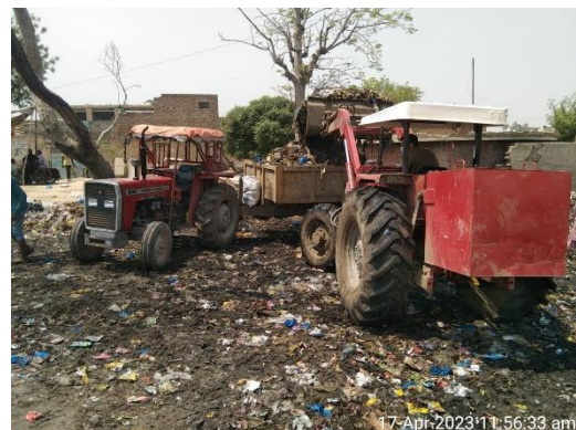
Figure 3: Working at Dump site
